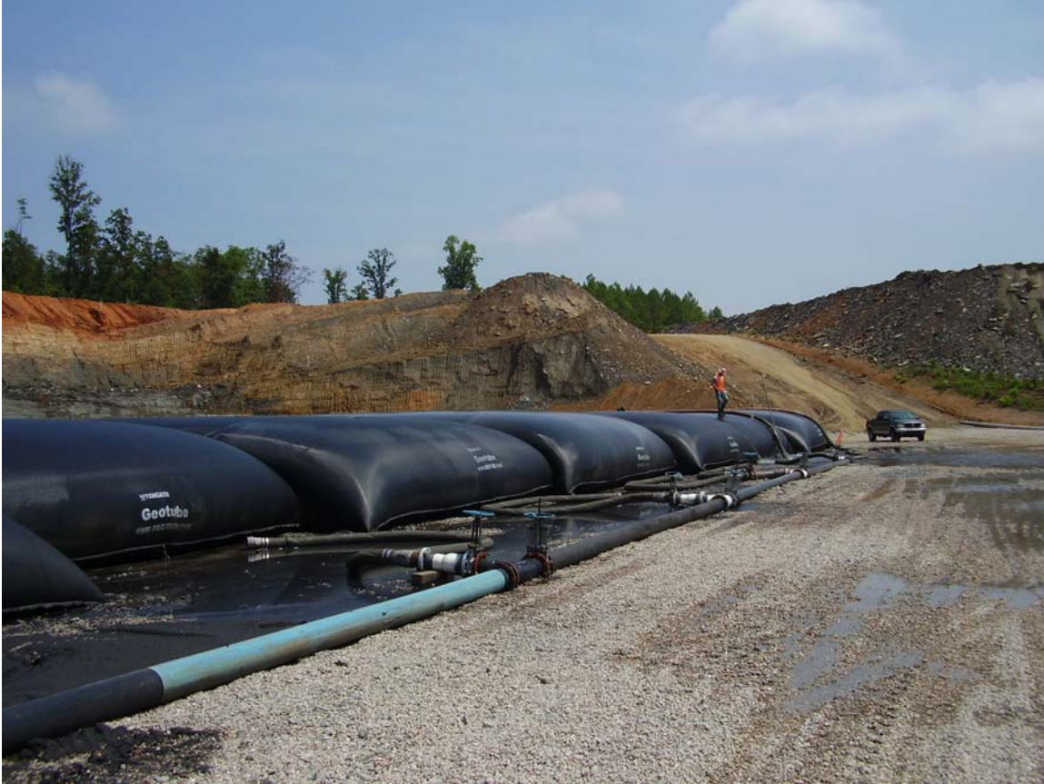
Figure 2 Example Site – Geotextile Tube Dewatering
