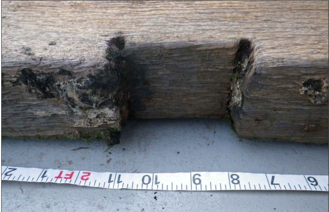
Figure 95: Limber hole of Timber 8 of A53. Note drilled holes in the corners, allowing for the rectangle to be sawn out (LCMM Collection).
