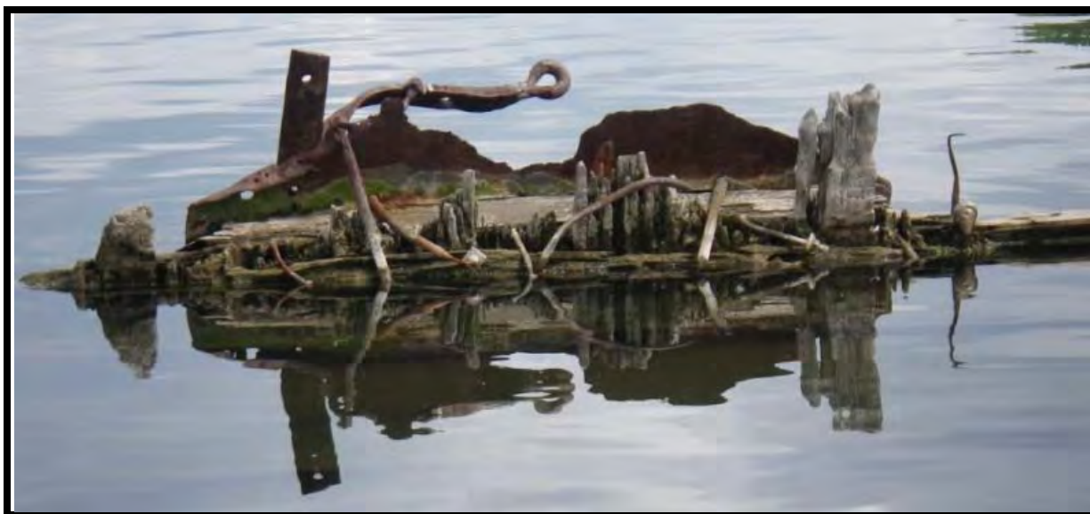
Figure 79: Inboard side of Anomaly A12's spud box (LCMM Collection).
