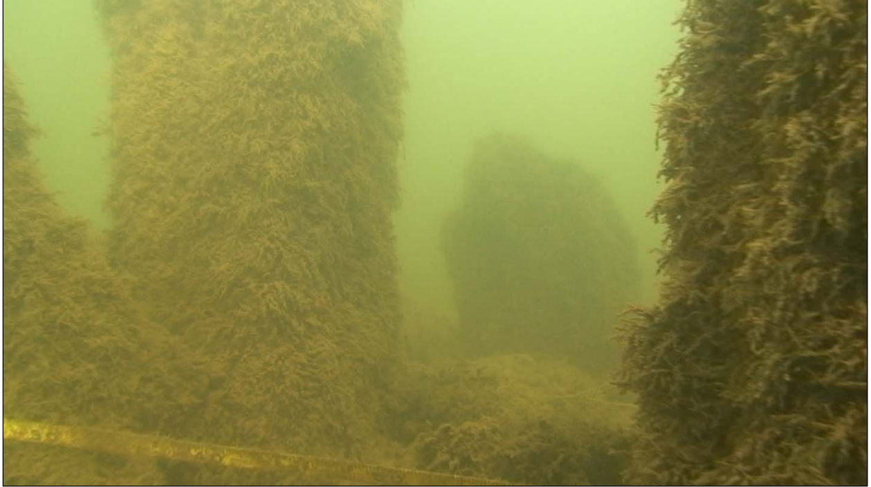
Figure 37: Vertical pilings at Salina Pier held back rip-rap, cobbles, or other fill (LCMM Collection).
