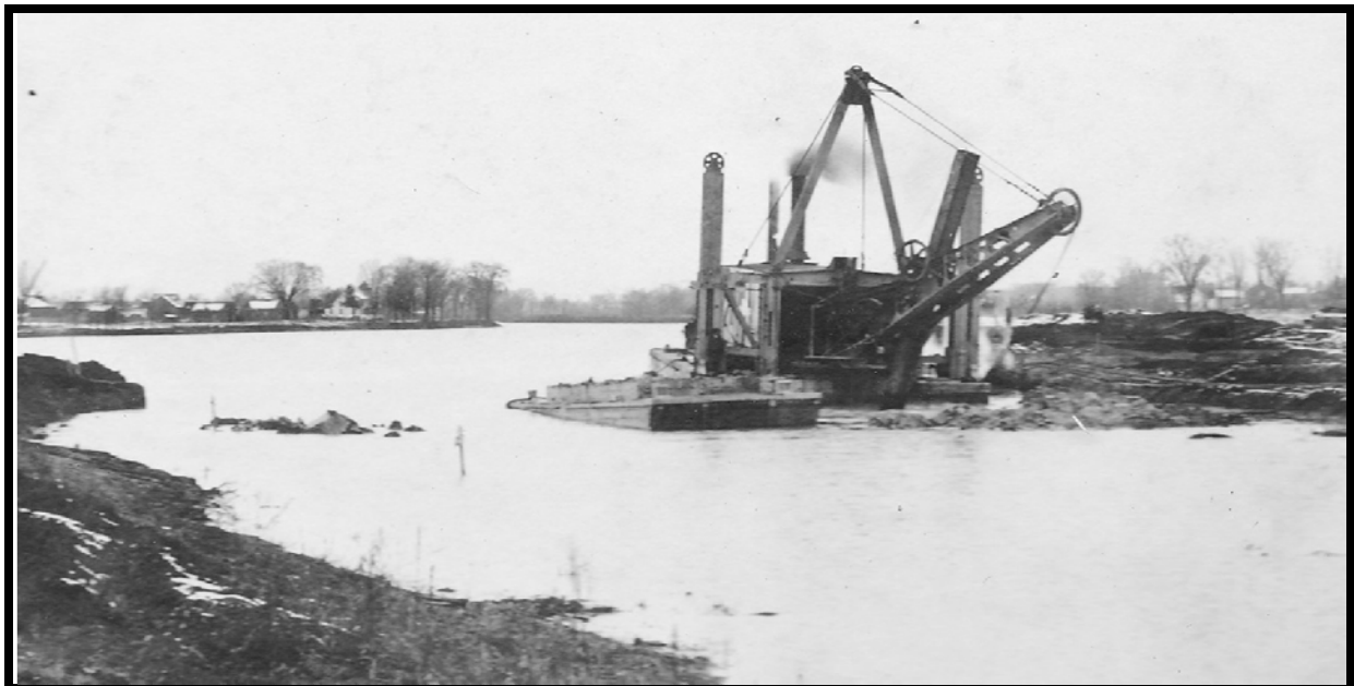
Figure 83: Photograph showing a bucket dredge with spuds excavating the barge canal in 1906 or 1907 with a dump scow in the foreground (LCMM Collection).
