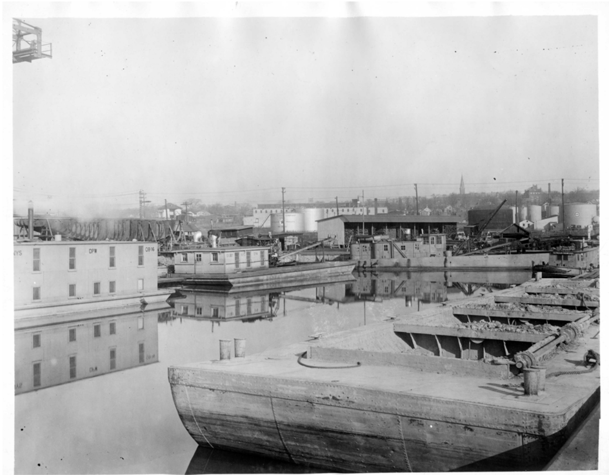
Figure 98: Dump Scow in Syracuse Inner Harbor 1914. This example displays composite construction instead of wooden construction but is otherwise similar to A4-1. (The Erie Canal Museum, Syracuse, NY, eriecanalmuseum.org )
