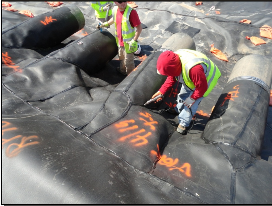
Photograph 9: The completed boots were non-destructively tested using the spark test method.
