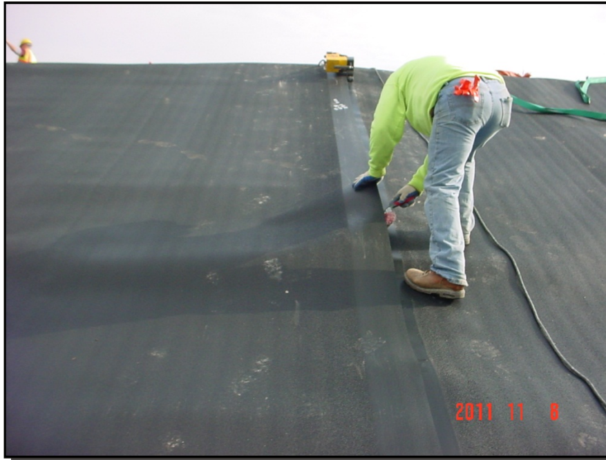
Photograph 3: Seams between adjacent panels were constructed using fusion welders. Welder operators cleaned the geomembrane along the overlap prior to seaming.
