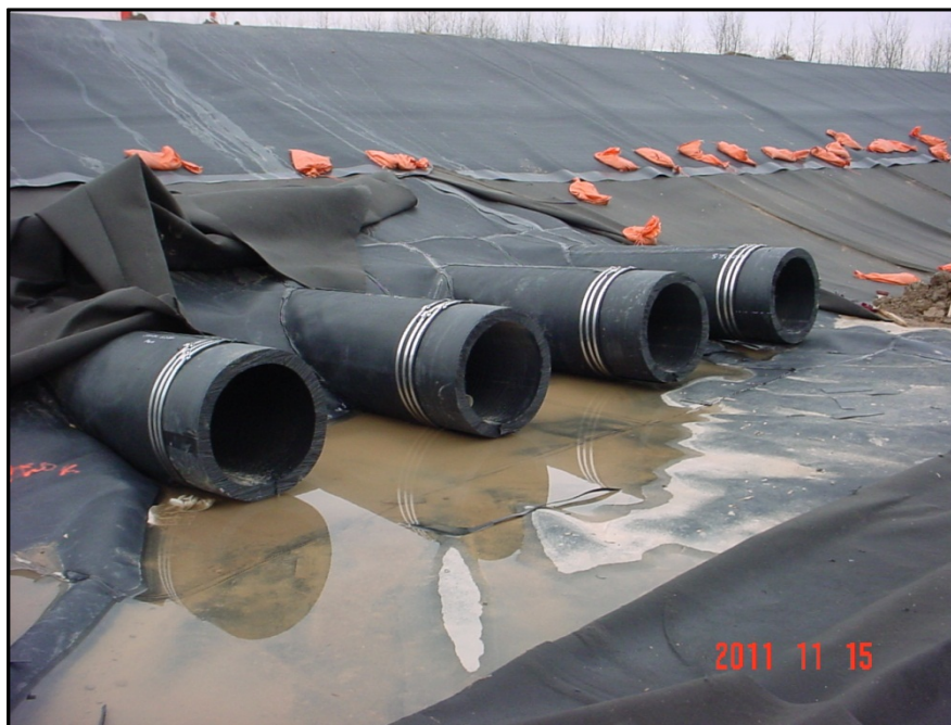
Photograph 8: Four 24-in dia. pipes penetrated the primary and secondary layers (secondary shown) of the liner system in each basin. Boots were constructed in the field and installed over the penetrations.
