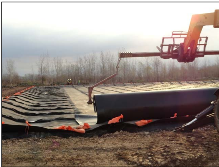
Photograph 16: Panels of the primary geomembrane layer were deployed from rolls suspended by a telehandler equipped with a spreader bar.
