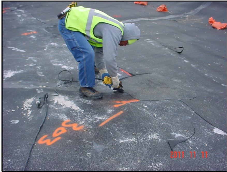
Photograph 5: Repairs to the geomembrane were heat bonded to the underlying material and the edges of the repair were abraded using an electric grinder.
