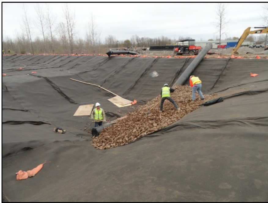
Photograph 14: Drainage gravel was placed over the riser pipe within the sump area as ballast and collection layer.
