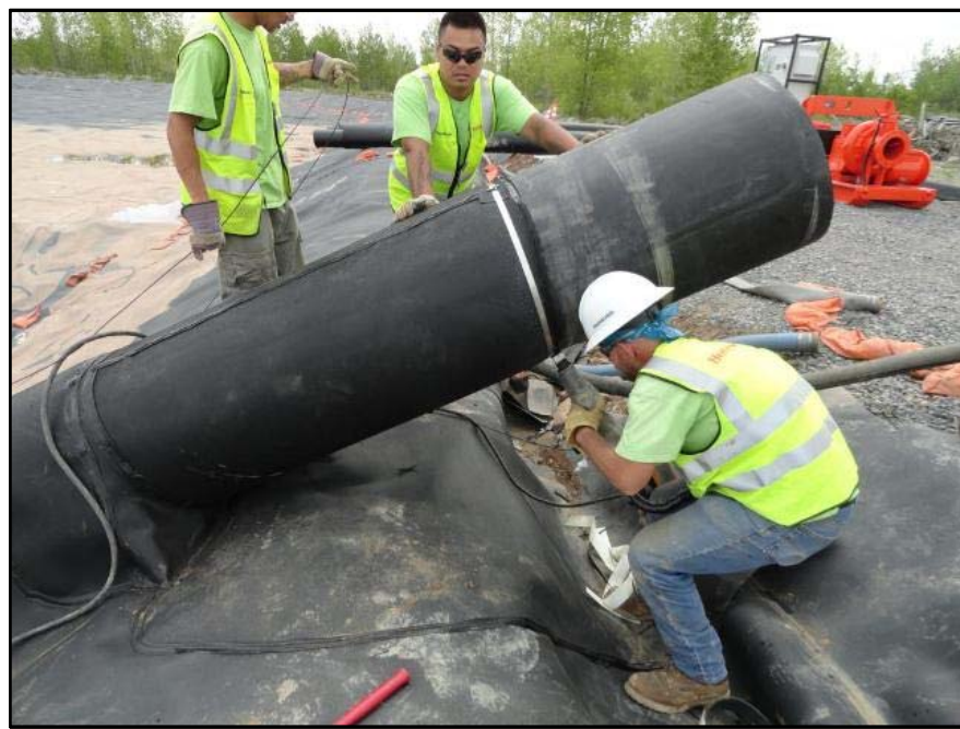
Photograph 22: Boots were installed where the side-slope riser of the leak detection system penetrates the primary liner.
