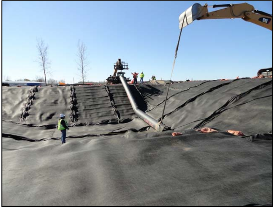
Photograph 13: A side-slope riser was installed within the sump of each basin between the primary and secondary layers as part of the leak detection system.
