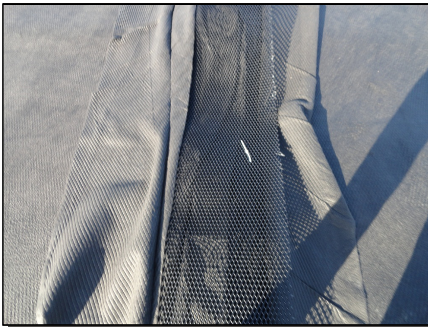
Photograph 11: The net component of adjacent geocomposite panels were connected using plastic ties.
