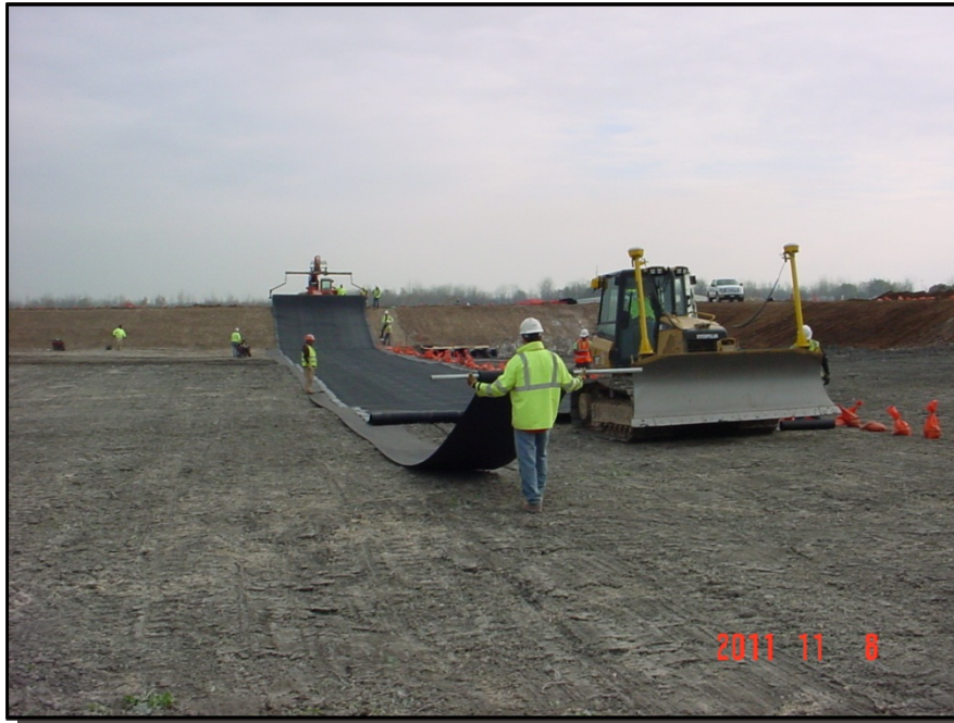
Photograph 1: Secondary layer panels of 60-mil thick HDPE geomembrane were deployed from rolls using a dozer. Roofing Felt was placed under edges of panels to minimize contact with the Solvay waste.
