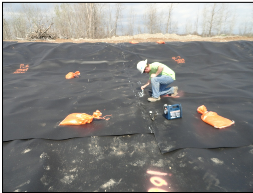
Photograph 4: Fusion welded seams were non-destructively tested using the air pressure method.
