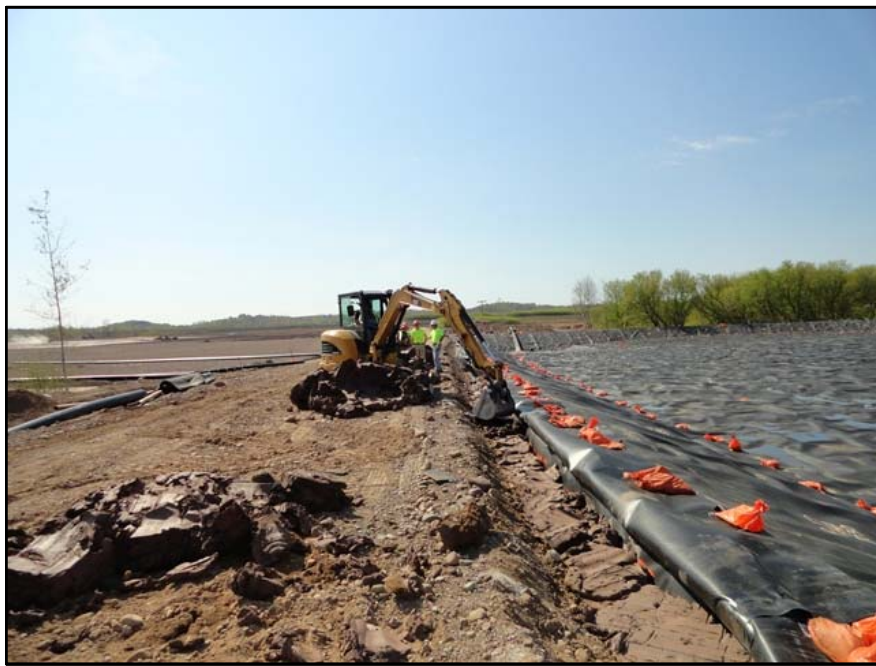
Photograph 20: The primary geomembrane was temporarily folded to facilitate installation of a LP soil plug in the anchor trench between the primary and secondary layers.
