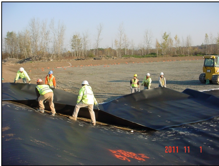
Photograph 2: Deployed panels were manually positioned to set panel overlap.
