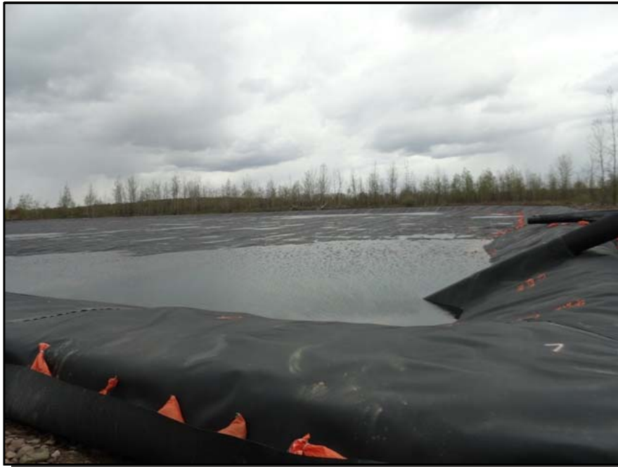
Photograph 19: A view of the completed geosynthetics prior to backfilling of the anchor trench.
