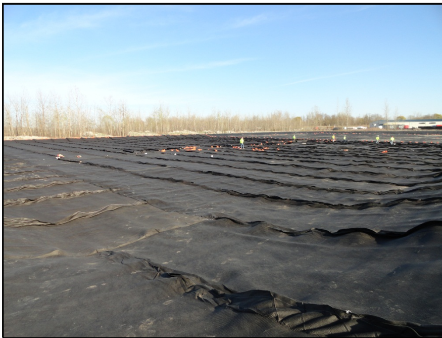
Photograph 10: Geocomposite was deployed over the secondary geomembrane layer.
