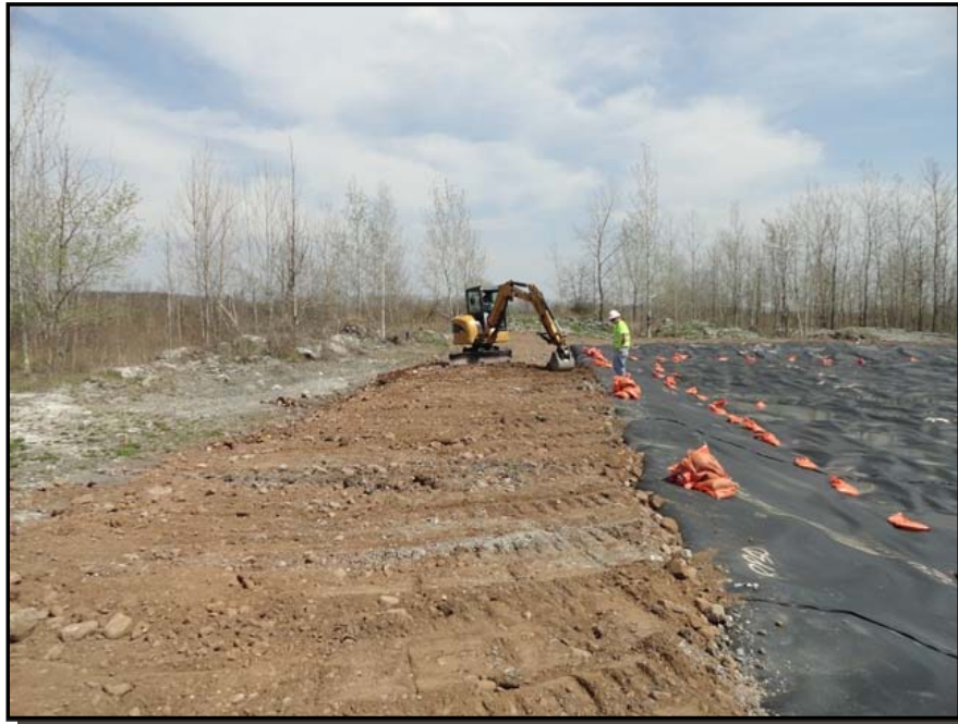
Photograph 21: The primary liner was then placed into the anchor trench and backfilling of the trench was completed.
