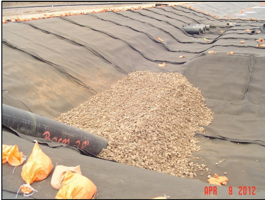
Photograph 15: A view of the riser structure upon completion of the Drainage Gravel placement.
