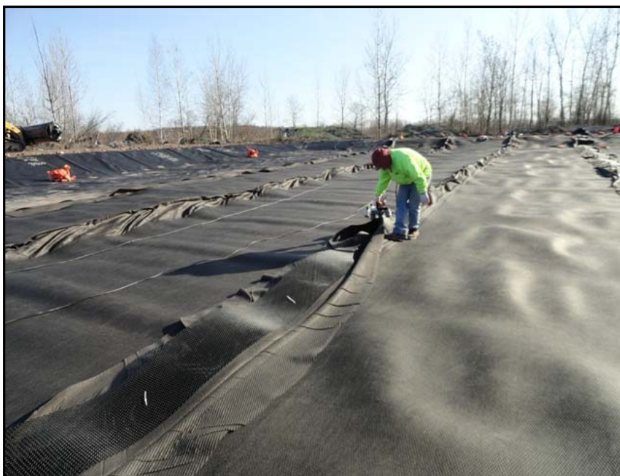
Photograph 12: The upper geotextile component of adjacent geocomposite panels was continuously sewn.
