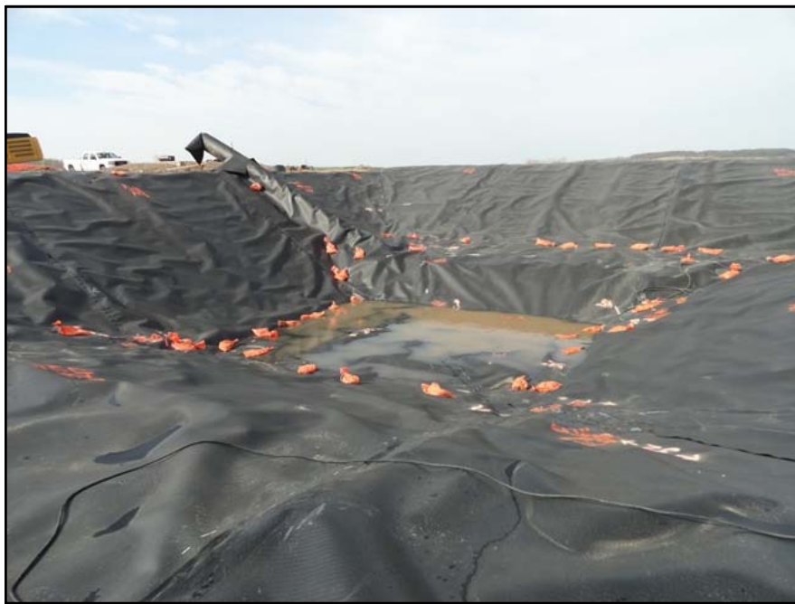
Photograph 18: The steps of seaming and repairing geomembrane outlined for the secondary layer were then implemented on the primary layer. A view of a completed basin sump is shown above.
