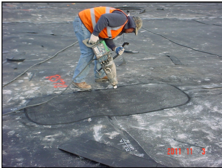
Photograph 6: Repairs to the geomembrane were extrusion welded.
