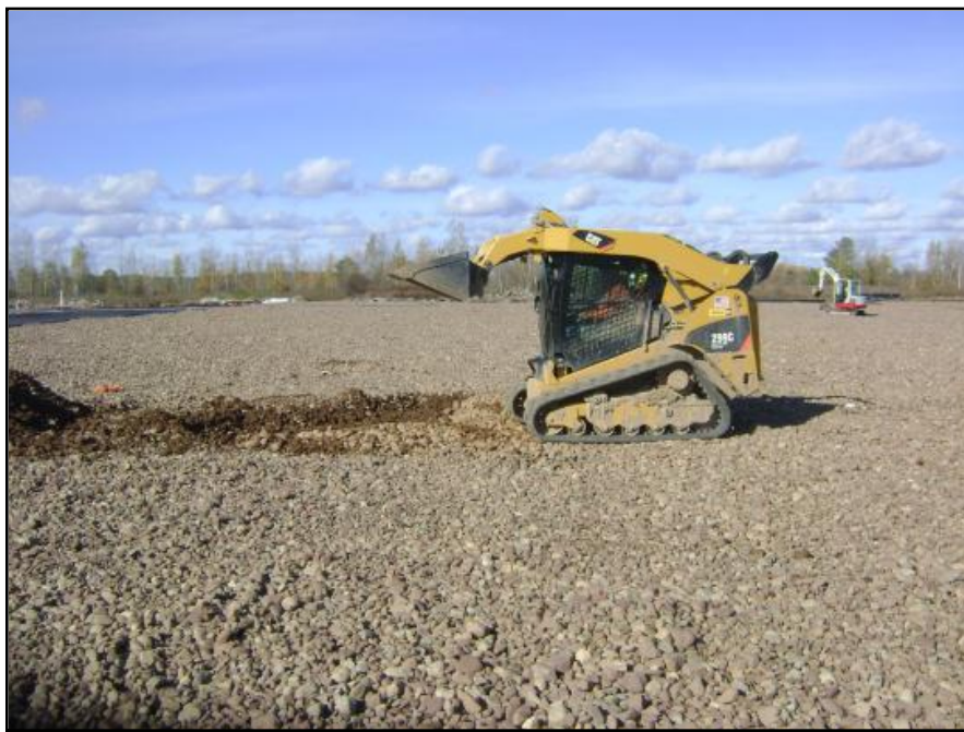
Photograph 34: Low-ground pressure equipment such as the Caterpillar 299 compact skid loader and Hitachi TB235 mini-excavator were used to remove areas of excessive fines.
