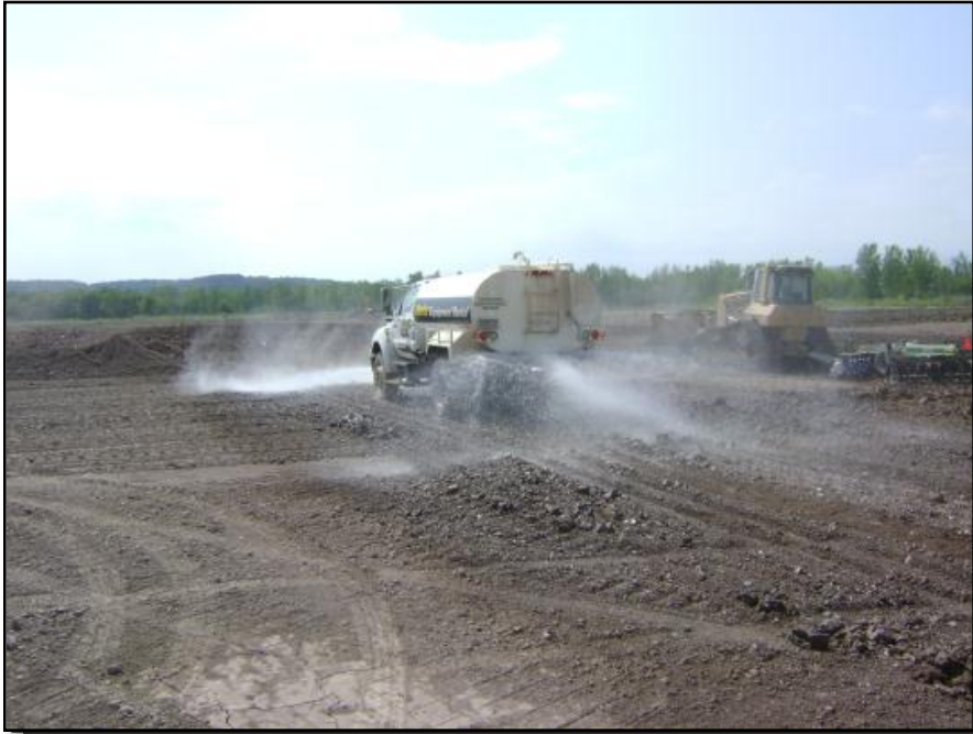
Photograph 11: Water was added to the low permeability soil, as needed. Occasionally, a tractor or bulldozer with a draw type harrow was used to condition the low permeability soil.
