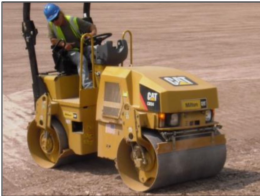
Photographs 13 and 14: In small areas, various compaction and surface preparations were performed. A Wacker 4614 or a Caterpillar CB24 rollers were used.
