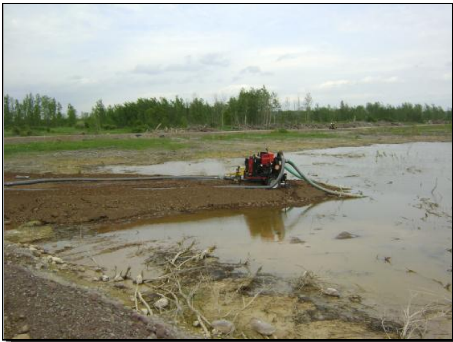
Photograph 6: Pumps were used during construction to remove stormwater from the work area.
