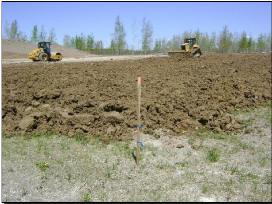
Photograph 9: Low permeability soil was delivered from two off-site sources, placed, and compacted to the grades defined in RFI No. 3 and Field Change Form (FCF) No. 3.
