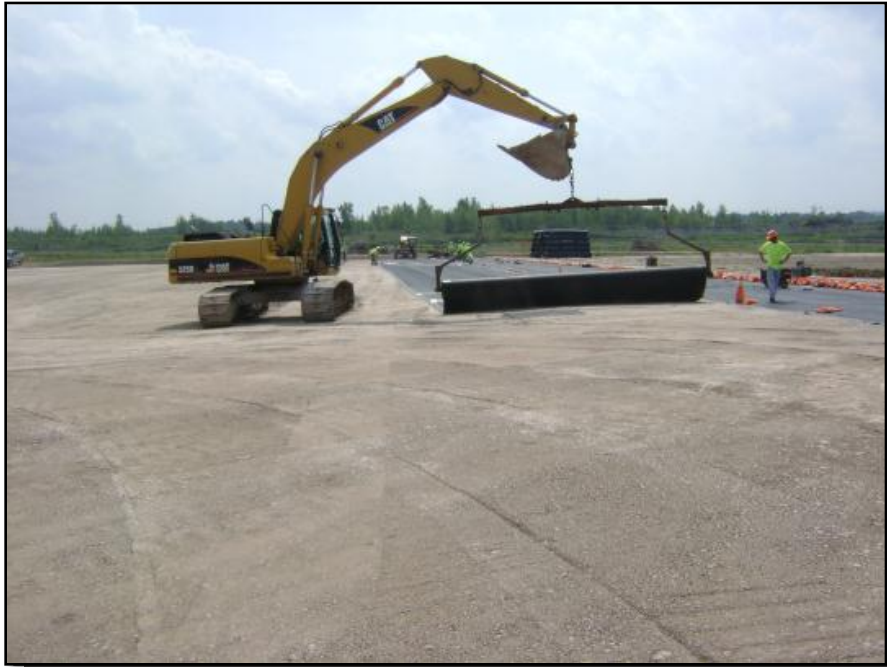
Photograph 25: Geomembrane rolls were deployed using a spreader bar attached to a piece of equipment, such as a Caterpillar 3250 excavator as shown above.
