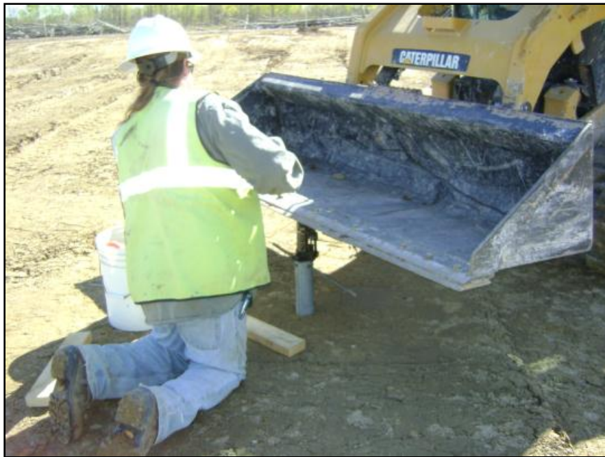
Photograph 16: CQA personnel verified the in-place moisture-density of the low permeability soil. Thin-walled (i.e. Shelby) tube samples were obtained from the upper lift, forwarded to an off-site testing laboratory, and tested to confirm the material met the hydraulic conductivity requirement.
