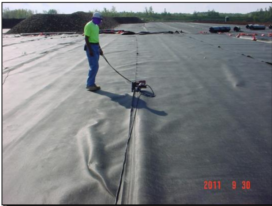
Photograph 30: A non-woven geotextile cushion was deployed over the geomembrane. Adjacent panels were thermally bonded using a single fusion welder.
