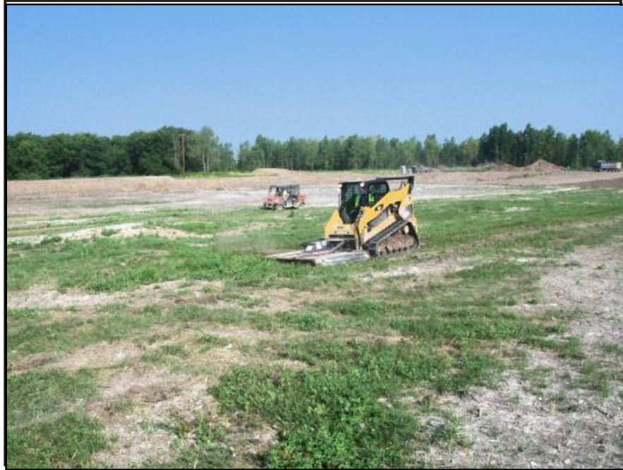
Photograph 3: Request for Information (RFI) No. 10 allowed the use of low-ground pressure bulldozers to strip the vegetation and debris. A skid loader with a brushcutter was used as well a bulldozer.
