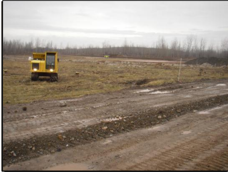
Photograph 1: The Sediment Consolidation Area (SCA) was cleared and partially grubbed prior to placement of engineered fill and low-permeability (LP) soil layer. In 2010, a LP soil test pad, shown in the background, was constructed.
