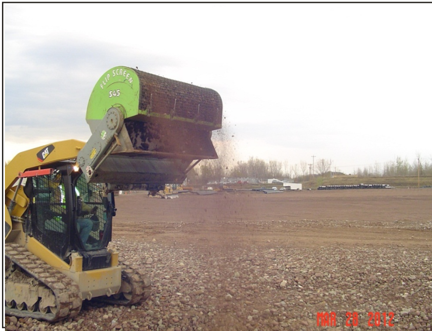
Photograph 38: In May 2012, a flip screener was used to further remediate areas of observed fines in the gravel drainage layer.
