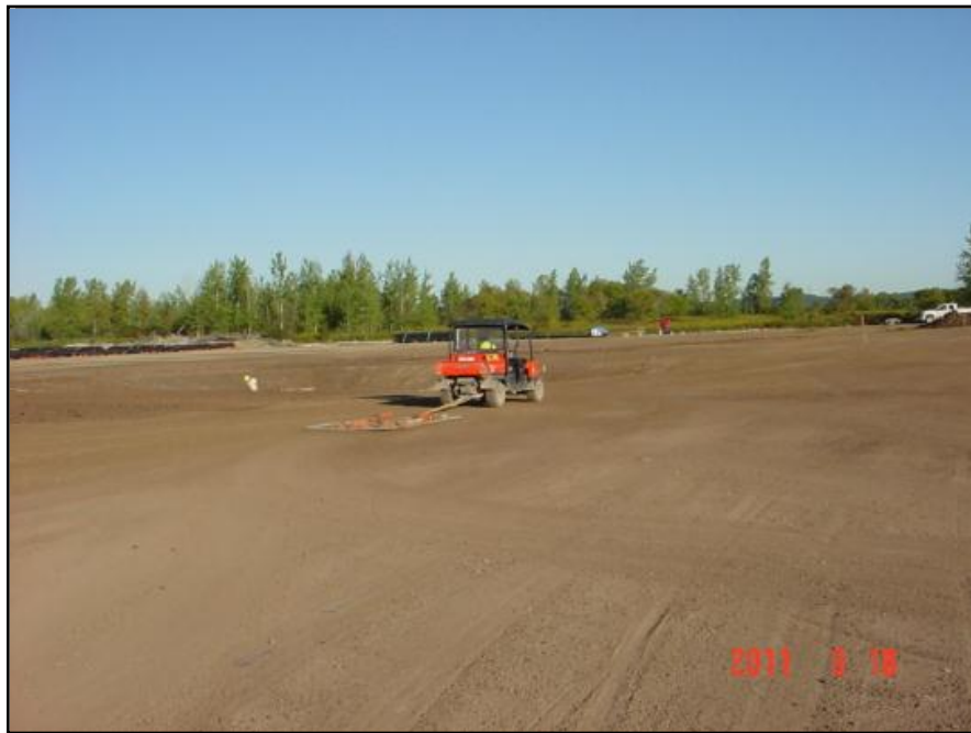
Photograph 12: Prior to geosynthetics installation, the surface of the low permeability layer was fine graded. Occasionally, an all-terrain vehicle pulling a weighted chain link fence was used to drag the surface, filling minor surface irregularities.
