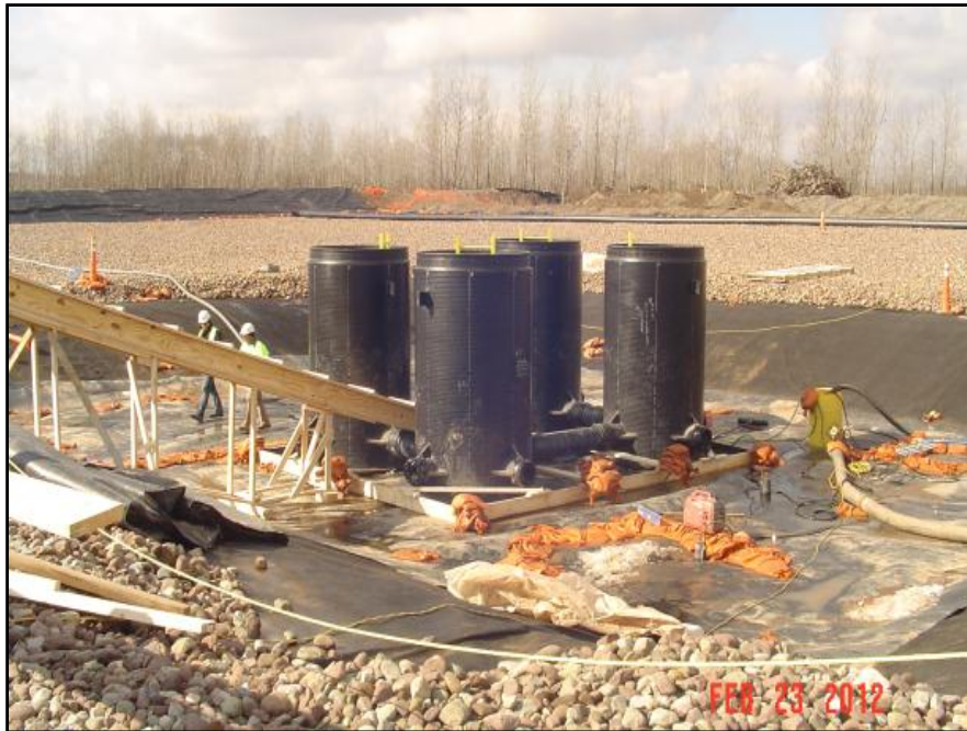
Photograph 39: In February 2012, polyethylene manholes were installed in the two sump areas. Concrete was placed around the four manholes. Gravel was later placed in the sump.
