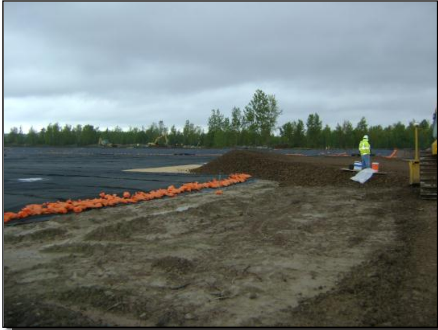
Photograph 31: Prior to placement of the gravel drainage layer, plywood was installed over the geosynthetics and gravel placed on top to establish access ramps.
