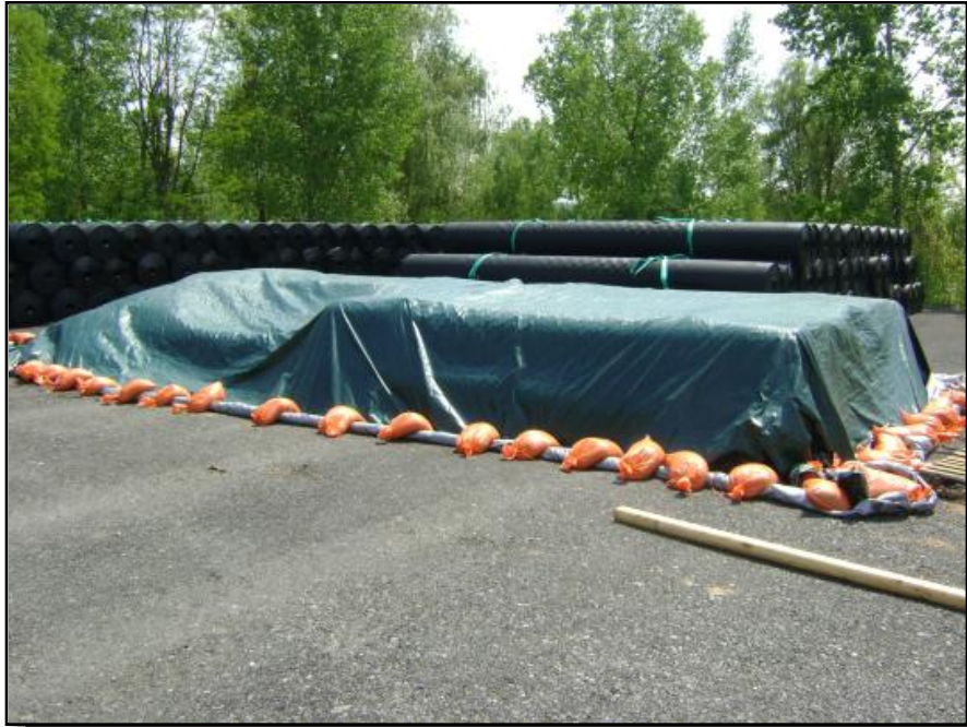
Photograph 23: Geosynthetic clay liner (GCL) was required in the sump areas. Rolls were stockpiled and covered next to the geomembrane rolls.
