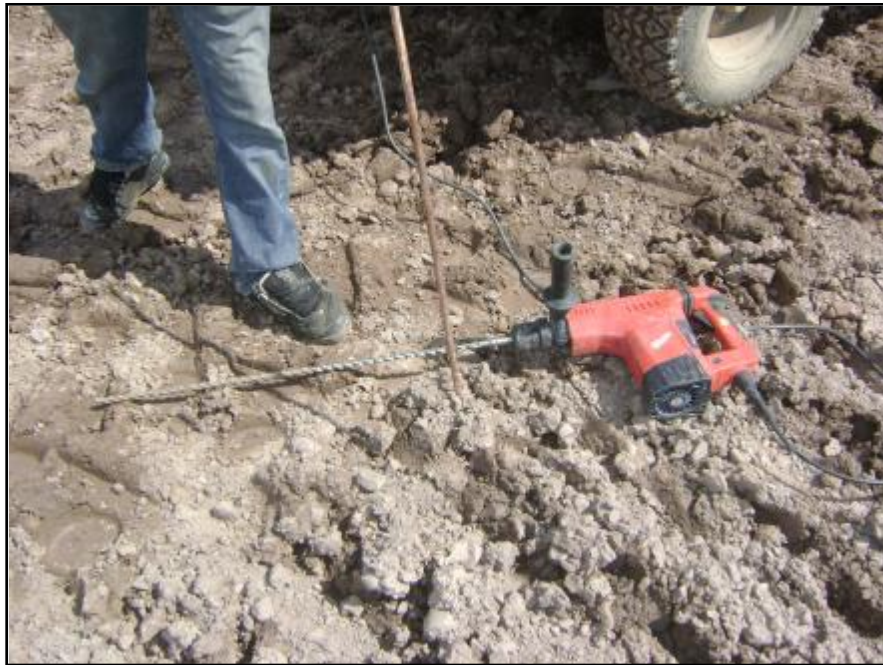
Photographs 17 and 18: Steel plates were installed within the Phase I sump corridor area. After low permeability placement, a drill was used to confirm that minimum clay thicknesses were achieved. Holes were backfilled using granular bentonite.
