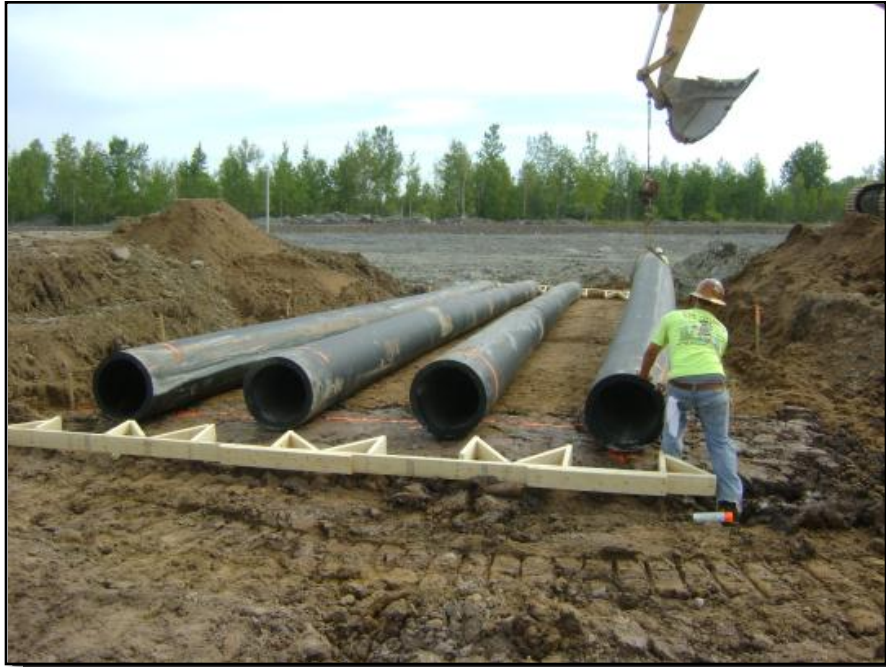
Photograph 19: Four 24-in dia. drainage pipes were installed through the eastern and western berms to connect to the Sediment Management System (SMS) stormwater basins.
