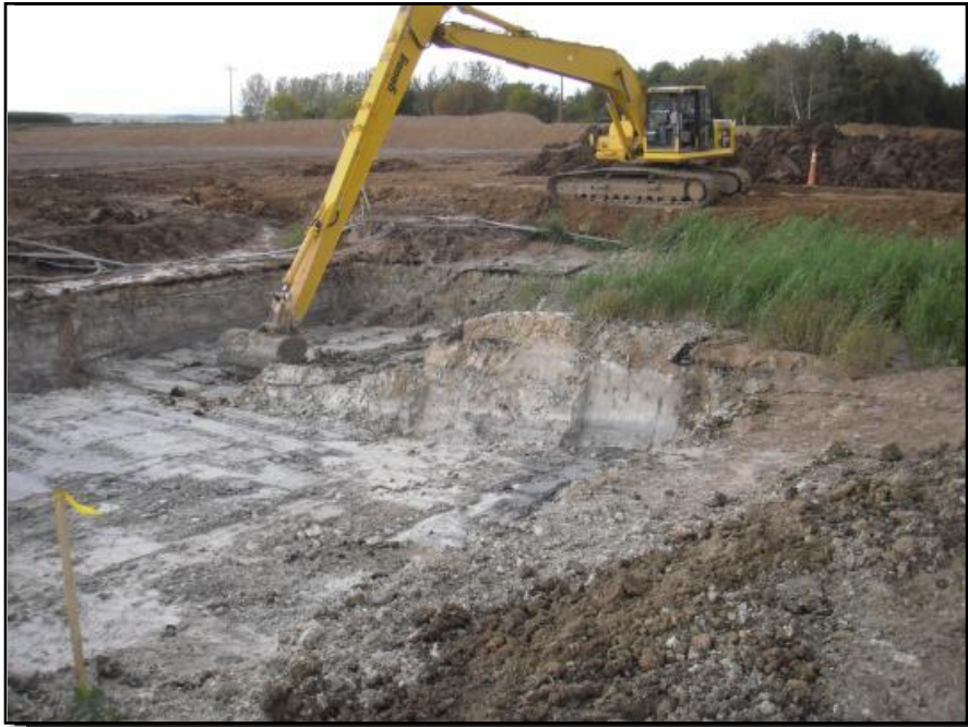
Photograph 21: Two sumps were excavated. The Solvay waste was re-located and the sump was lined with low permeability soil.
