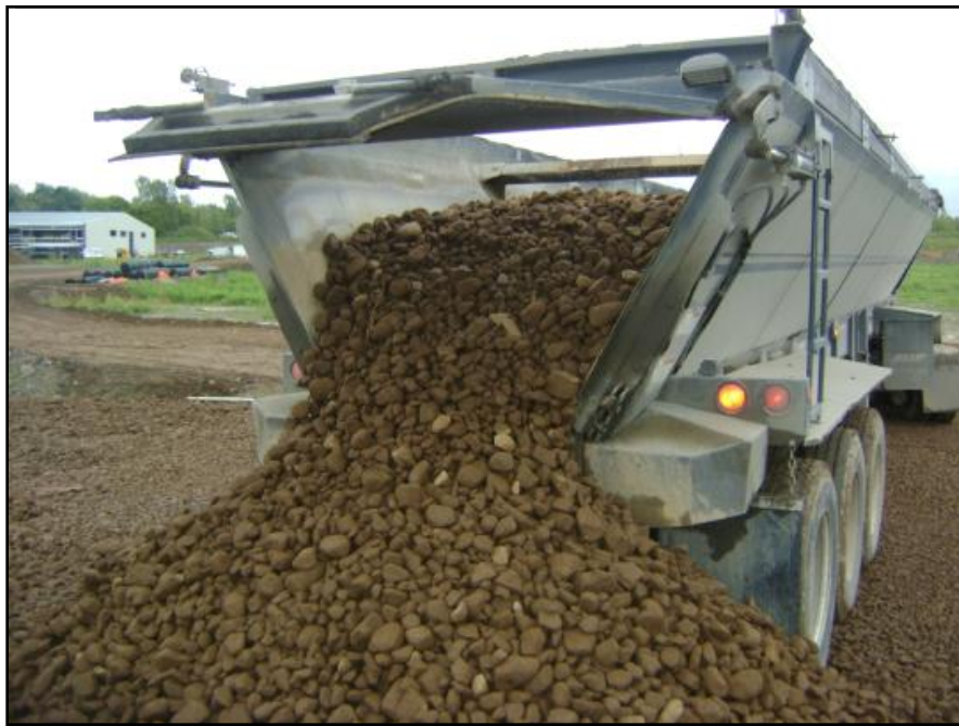
Photograph 32: Gravel was delivered primarily from the Granby source using live bottom trucks.
