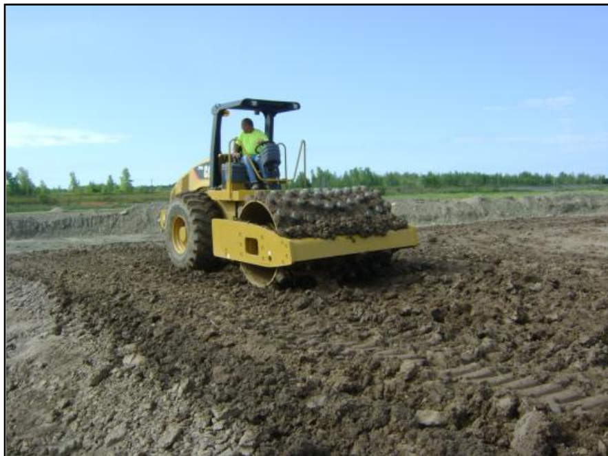
Photograph 10: Lifts of low permeability soil were compacted by a smooth drum or, as shown above, a pad-foot roller.
