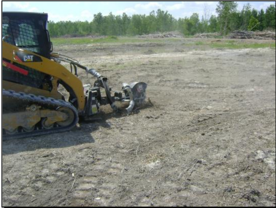
Photograph 5: Stumps were ground below the subgrade surface using a grinder. The prepared subgrade was observed and approved by NYSDEC and CQA personnel before placement low permeability layer.
