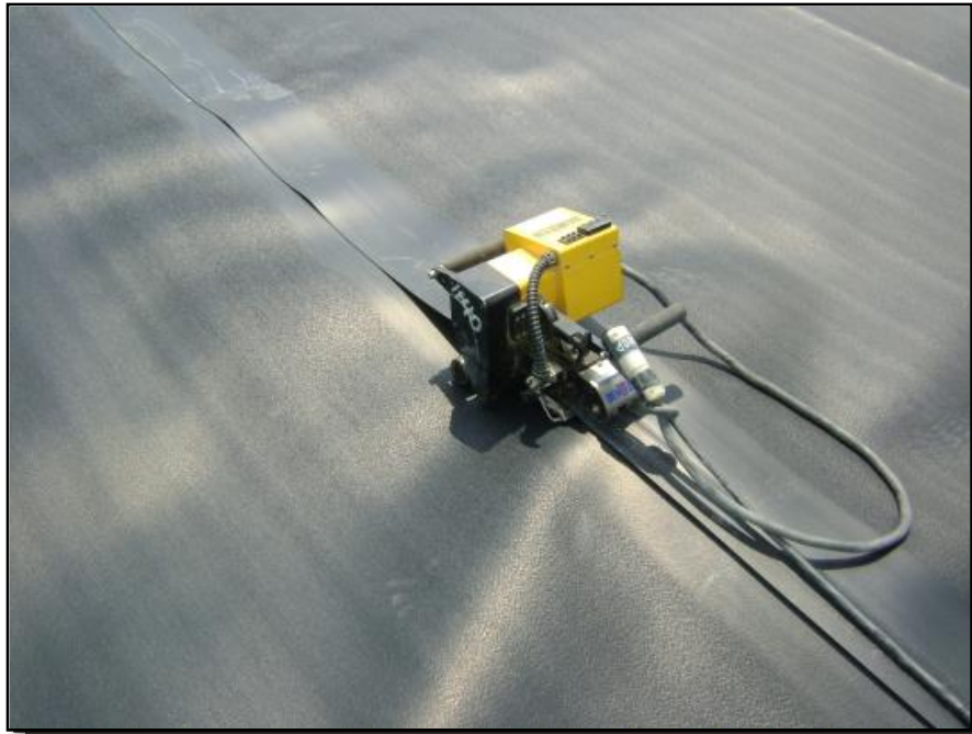
Photograph 27: A dual track fusion welder used to seam geomembrane panels together.
