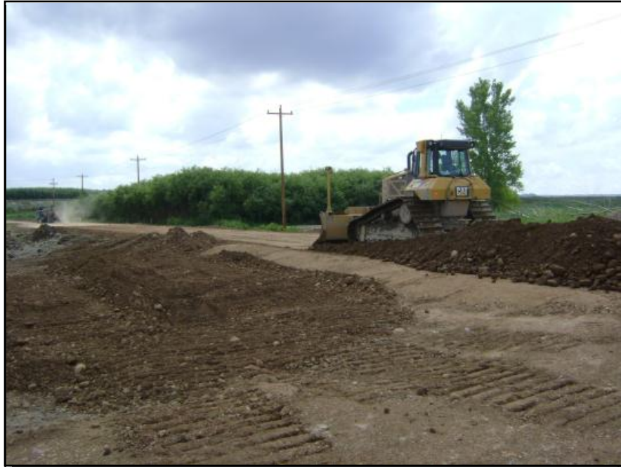
Photograph 7: Off-site engineered fill was used to construct perimeter berms. A bulldozer was used to spread the soil in lifts that were densified with a compactor. In-place compaction tests were performed by the contractor's laboratory or by CQA personnel after mobilization.
