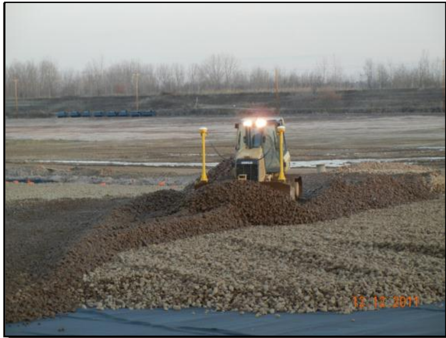
Photograph 33: Low-ground pressure dozers were used to place the gravel in a single lift.
