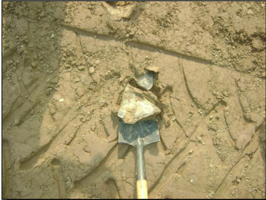
Photograph 15: Visible rocks were removed manually from the low permeability soil layer prior to geomembrane deployment.
