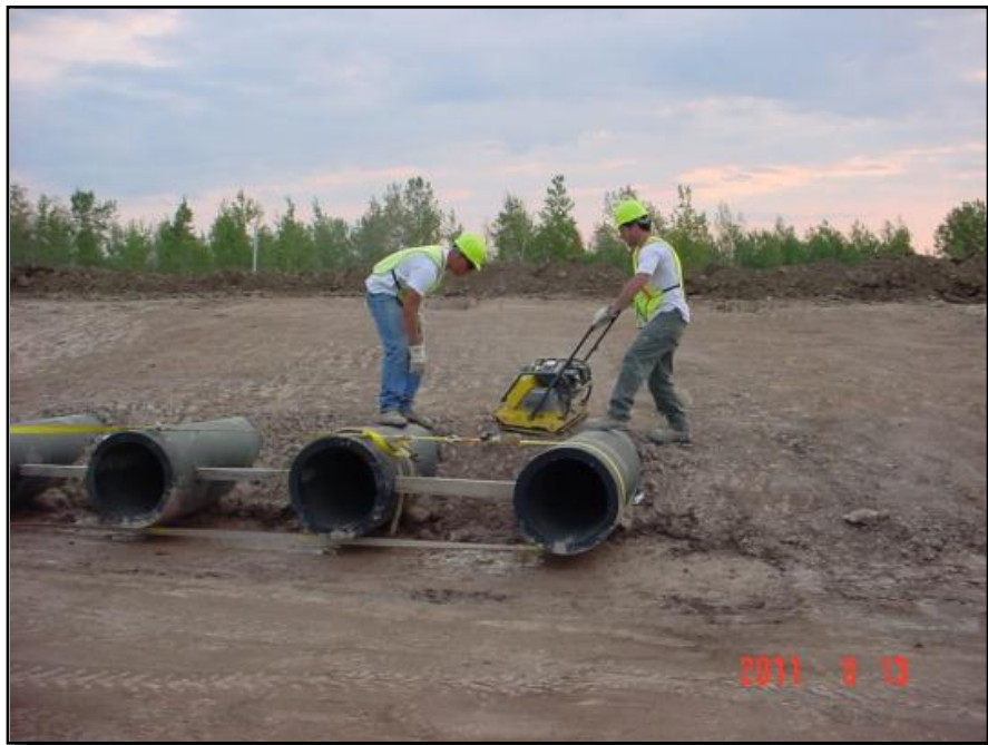
Photograph 20: Pipe bedding material was manually compacted. Engineered fill above the bedding material was compacted using a walk-behind compactor plate.
