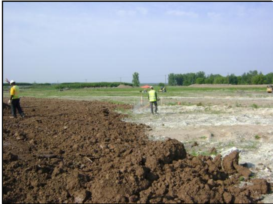
Photograph 8: The initial 12-in thick lift of low permeability soil was placed over the approved cleared area. This lift was considered a bridge lift.
