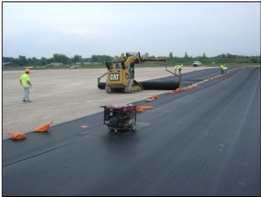
Photograph 26: A skid loader was also used to deploy geomembrane rolls. Panels were manually positioned before being welded. A wire was deployed under geomembrane panels to facilitate the leak location survey.
