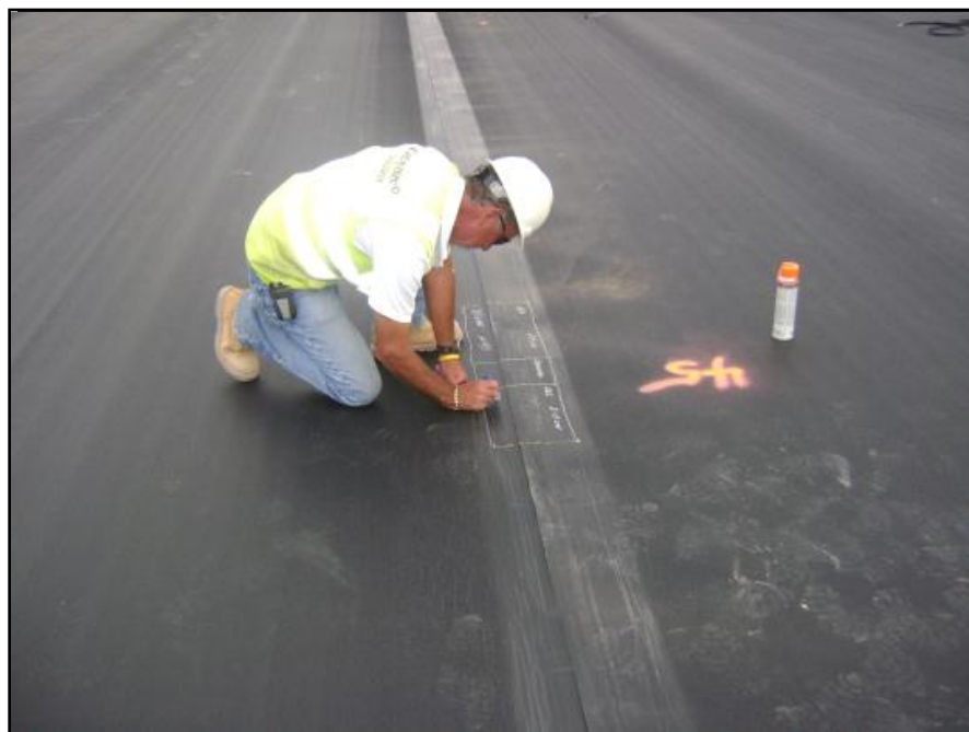
Photograph 28: CQA personnel monitored the geosynthetics installation and marked out destructive seam samples, as shown above. The samples were removed and tested to confirm the strength of the welds. The installer performed non-destructive test to confirm the integrity of the seams.
