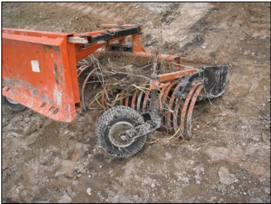
Photograph 4: A landscape rake was also used to remove roots and debris from the subgrade surface.
