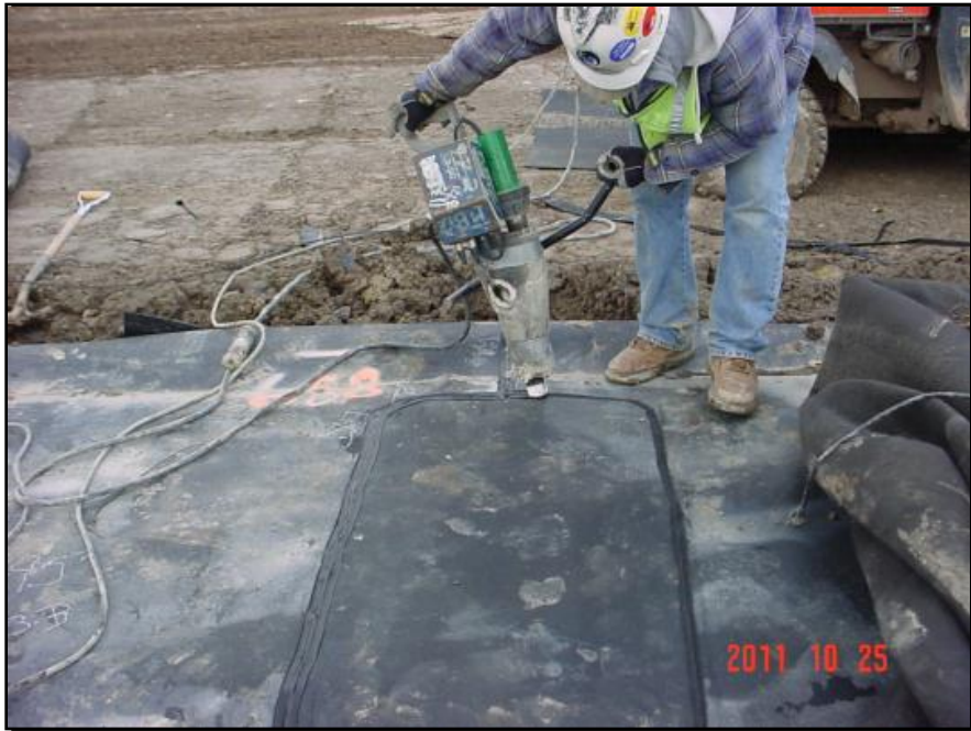
Photograph 29: The installer repaired the geomembrane liner by extrusion welding patches, as shown above.
