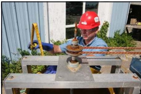
Record level in mix tank and subtract amount from previous volume to attain gallons of slurry processed in 1st phase fill
