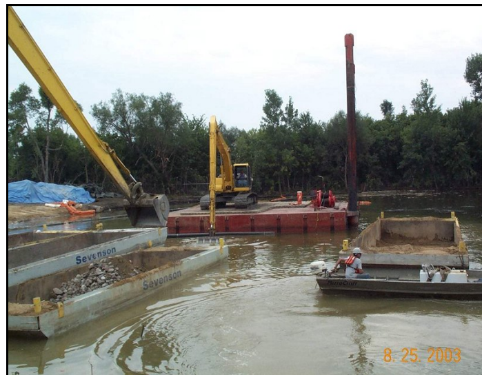
Figure 4. Mechanical Placement of Rock Cap Materials from a Shallow Draft Barge
