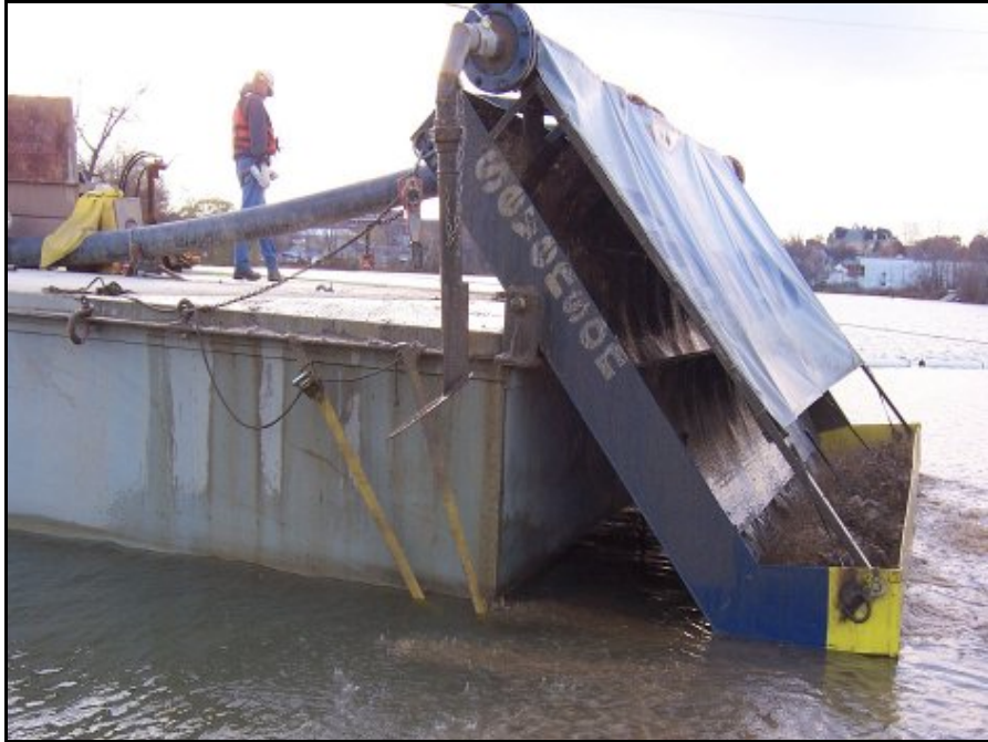
Figure 1. SES Spreader Barge System Placing Sand Cap Materials.
