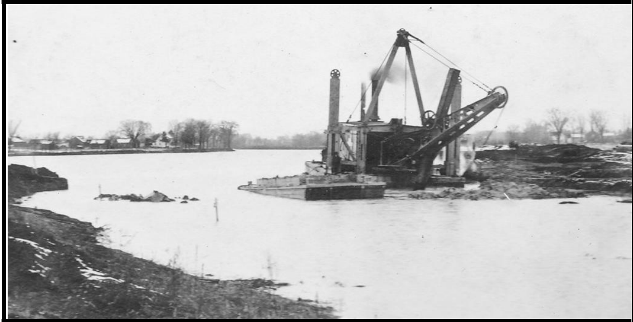
Figure 22. Photograph showing a bucket dredge with spuds excavating the barge canal in 1906 or 1907 with a dump scow in the foreground (LCMM Collection)
