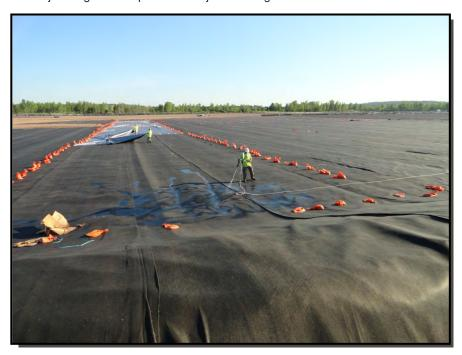
**Photograph 22:** The slopes of Phase II were leak tested using the water lance method prior to installation of a sacrificial geomembrane layer.
