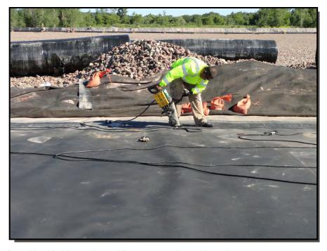
Photograph 18: Hand-held extrusion welders were used to weld repairs.
