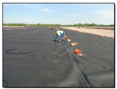
Photograph 15: Seams between adjacent geomembrane panels were constructed using fusion welding equipment.
