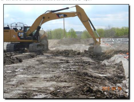
**Photograph 6:** An excavator was used to remove overburden along the Phase I tie-in.
