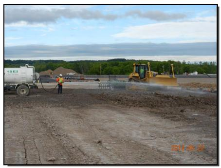
Photograph 5: Water was added to the scarified surface, as necessary, to promote adhesion between the lifts of LP soil and to maintain the moisture content of the LP layer.
