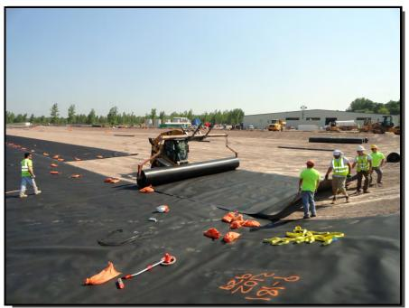
Photograph 12: A compact track loader was used to deploy panels from rolls of 60-mil thick HDPE geomembrane.
