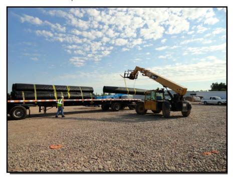
**Photograph 10:** Additional geomembrane rolls were delivered to the site during construction of Phase II. The material was unloaded and stockpiled on-site using a telehandler.
