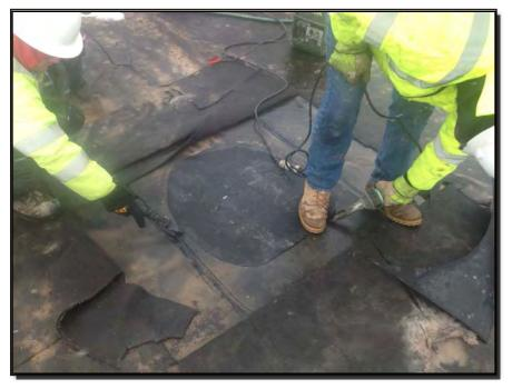
Photograph 32: Chenango mobilized to the SCA on 3 April 2013 to repair the hole at the former location of inclinometer SI-G1 by extrusion welding a patch. Parsons placed the gravel drainage layer after repairs were completed.
