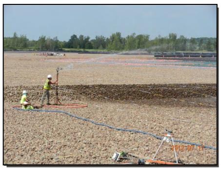
**Photograph 28:** Sprinklers were used to apply water to the installed drainage gravel layer and underlying geosynthetics to facilitate electrical leak location surveying (ELLS).
