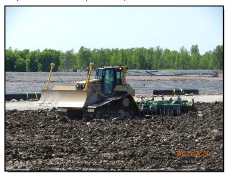
**Photograph 2:** A dozer and draw-type harrow was used to homogenize placed lifts of LP soil.
