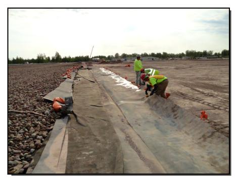
**Photograph 11:** The Phase I geomembrane was unfolded over the completed LP soil layer prior to welding a connection to the Phase II geomembrane.
