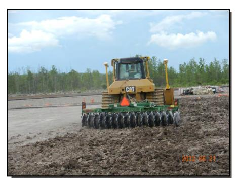
**Photograph 4:** The surface of LP soil lifts were scarified approximately 2-in deep prior to placement of subsequent lift.
