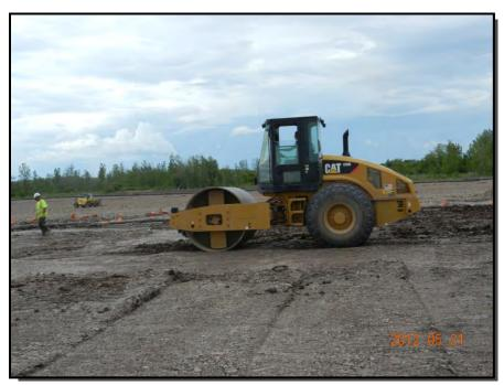
**Photograph 3:** Placed lifts of LP soil were compacted using a CAT CS-56 vibratory roller.
