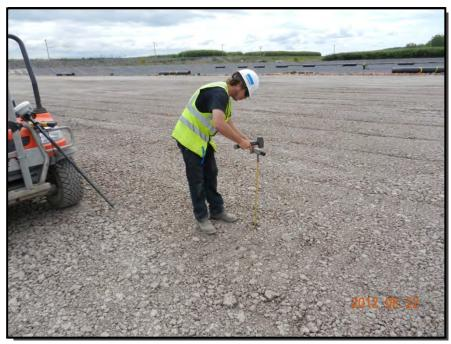
**Photograph 9:** LP layer thickness verification was performed by Parsons using either a driven probe rod (shown) or a drill bit to contact steel plates.
