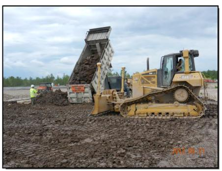
**Photograph 1:** The Phase II LP soil material was placed using Caterpillar D6N dozers equipped with GPS guidance systems. The material was placed in multiple lifts to achieve a minimum thickness of 1-ft.
