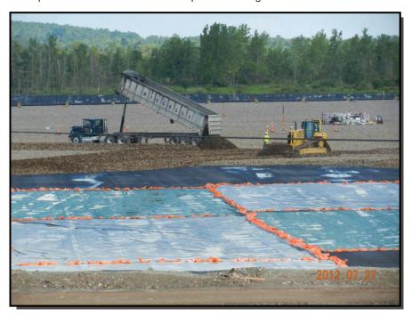
**Photograph 26:** Two foot thick access roads were established inside the Phase II area on which trucks transporting drainage gravel used. After unloading, gravel was placed to a thickness of 1 ft using Caterpillar D6N LGP dozers.
