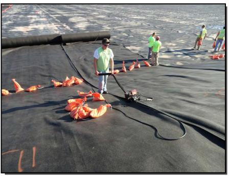
**Photograph 21:** A non-woven geotextile cushion (24 oz/syd) was deployed over the installed geomembrane. Adjacent geotextile panels were joined using a fusion welder.
