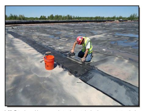
**Photograph 20:** Extrusion welds were non-destructive tested using the vacuum test method.
