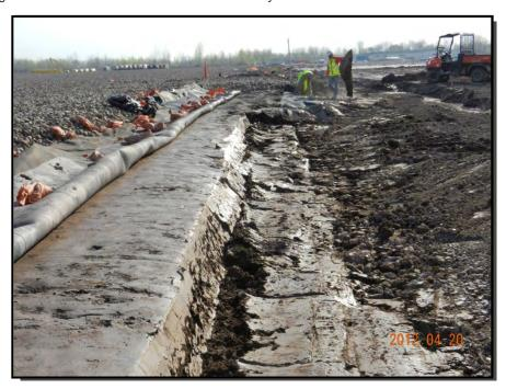
**Photograph 8:** The LP soil layer in Phase I was trimmed to a shear face to ensure the minimum layer thickness was achieved along the tie-in.
