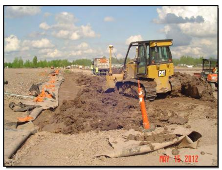
**Photograph 7:** The geomembrane in Phase I was rolled back and ballasted to facilitate access to the underlying LP soil to allow the Phase II LP soil to be keyed in.
