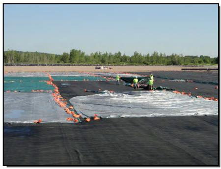
**Photograph 25:** Temporary tarpaulins were used to cover areas of installed geotextile to minimize UV exposure. the tarpaulins were re-located with the placement of gravel.
