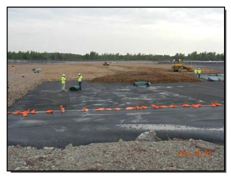
**Photograph 27:** The tarpaulins covering the geotextile were removed as drainage gravel placement progressed.
