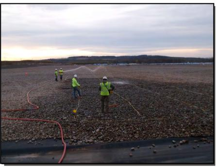
**Photograph 29:** The ELLS was performed using the dipole method. The locations of data anomalies were excavated. Located holes were repaired, the gravel was reinstalled, and the area retested.
