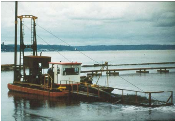
Cap Placement Using Clean Sand
