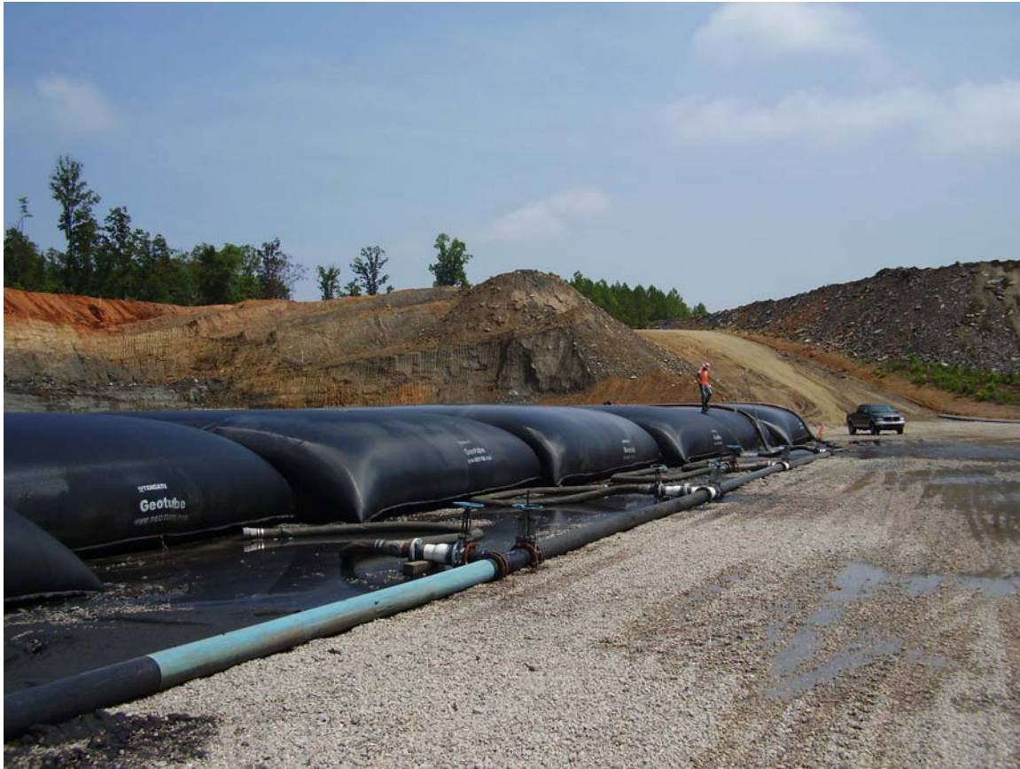
Figure 2 Example Site – Geotextile Tube Dewatering
