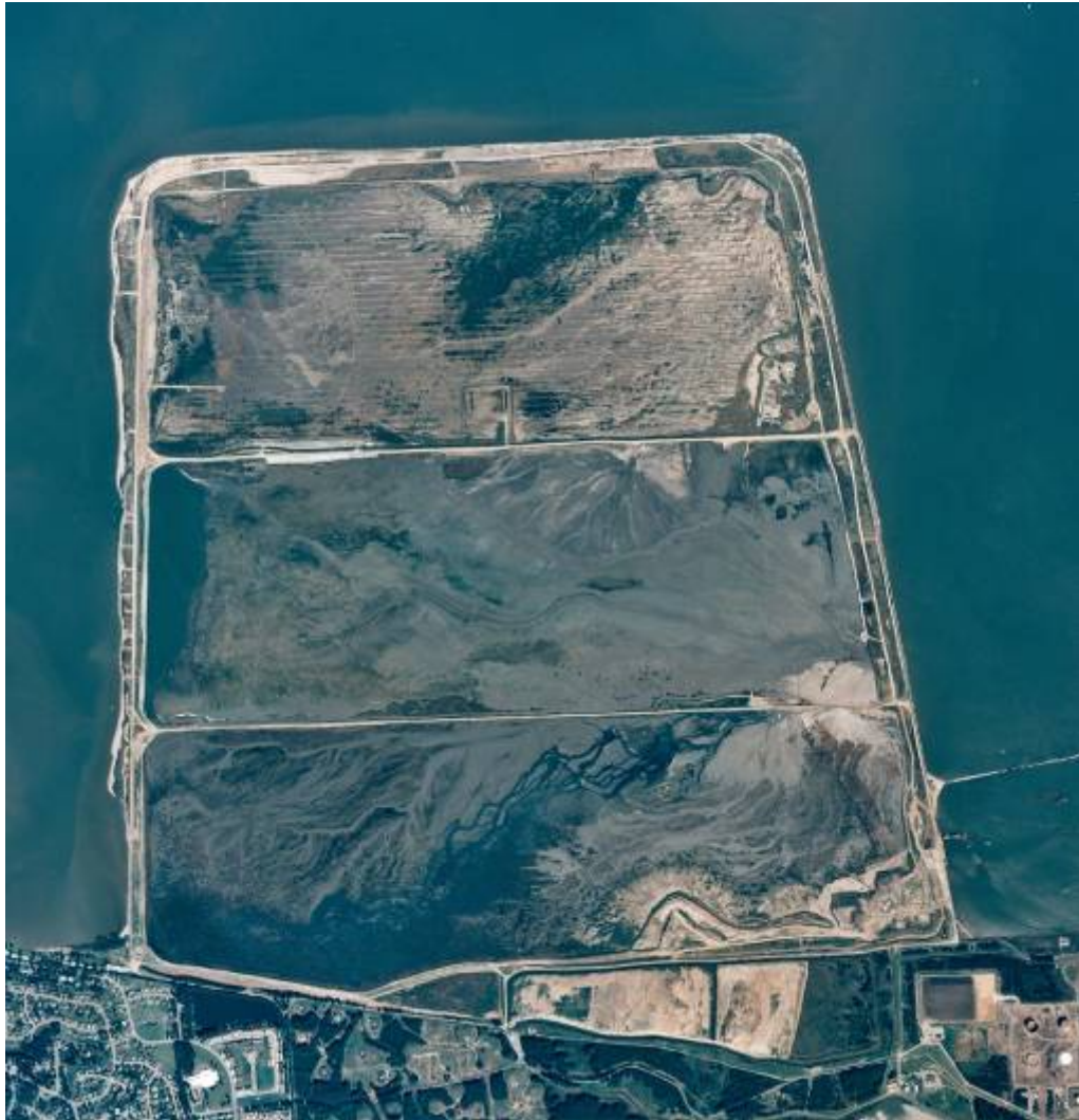
Figure 1 Example Site – Settling Basin
