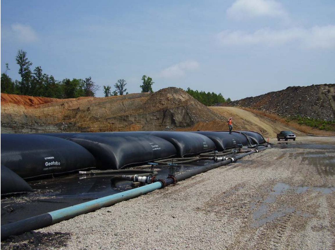
Figure 2 Example Site – Geotextile Tube Dewatering
