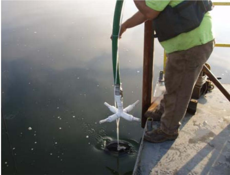
Diffuser before being submerged.
