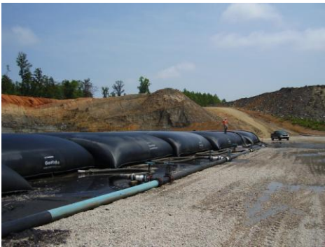
Geotextile tube dewatering operation
