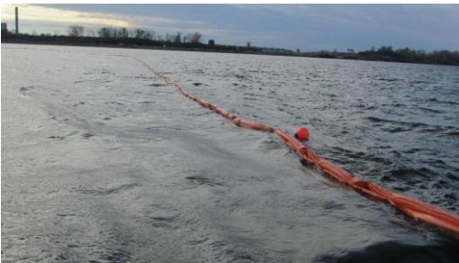
Silt curtain being deployed on Onondaga Lake.
