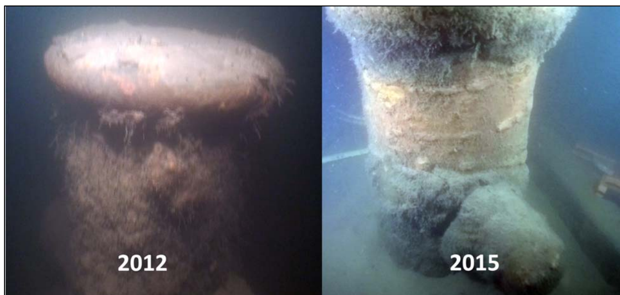
Figure 19: Comparison of bollard condition in 2012 vs. 2015 (LCMM Collection)
