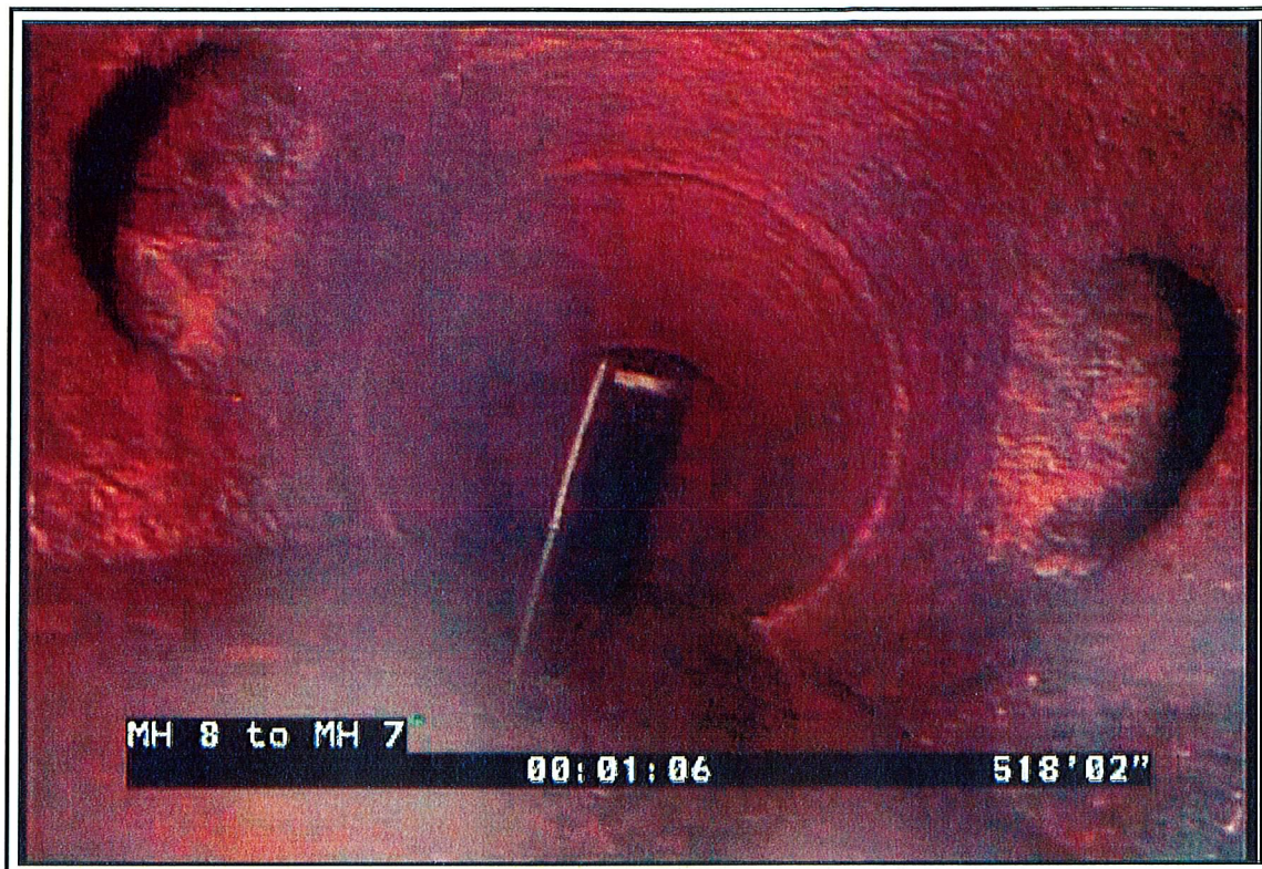
Photo 1: Image of lateral connections and plug valve at MH-7 in 30-Inch Force Main.
