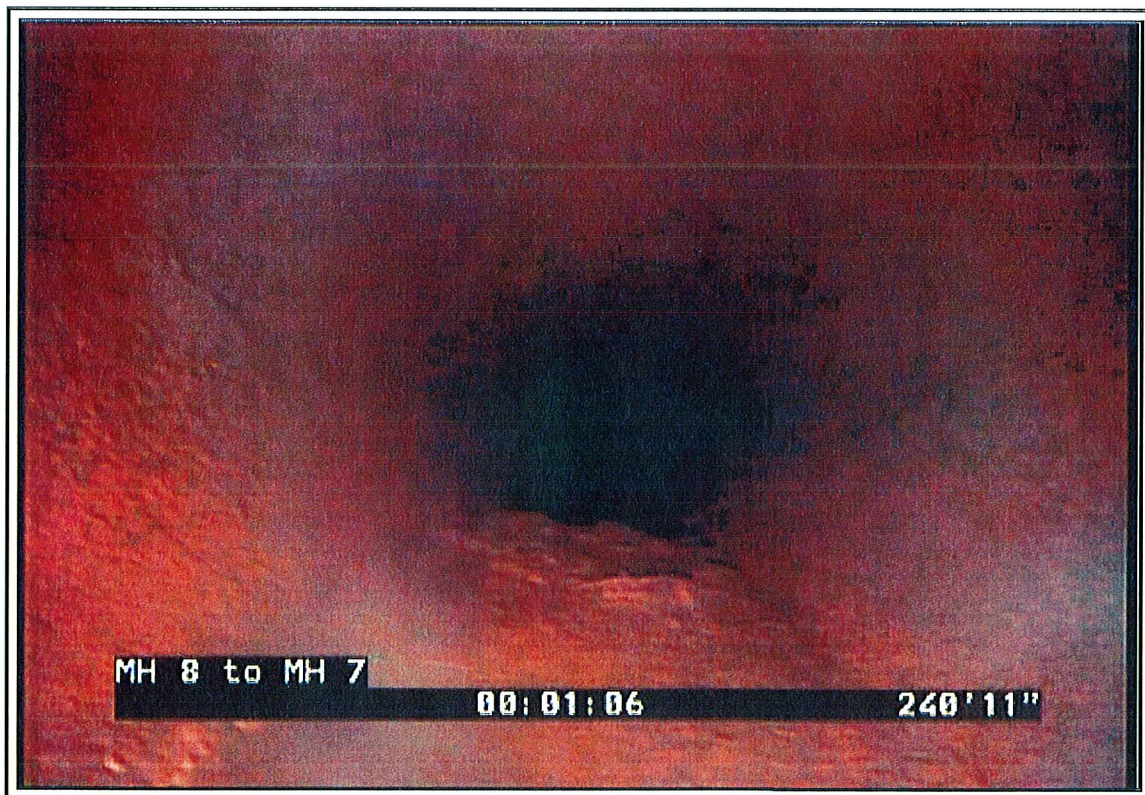
Photo 4: Section of the 30-Inch Force Main in the direction of MH-7 taken 240'-11" from MH-8. This section has standing water after pumps were shut off.
