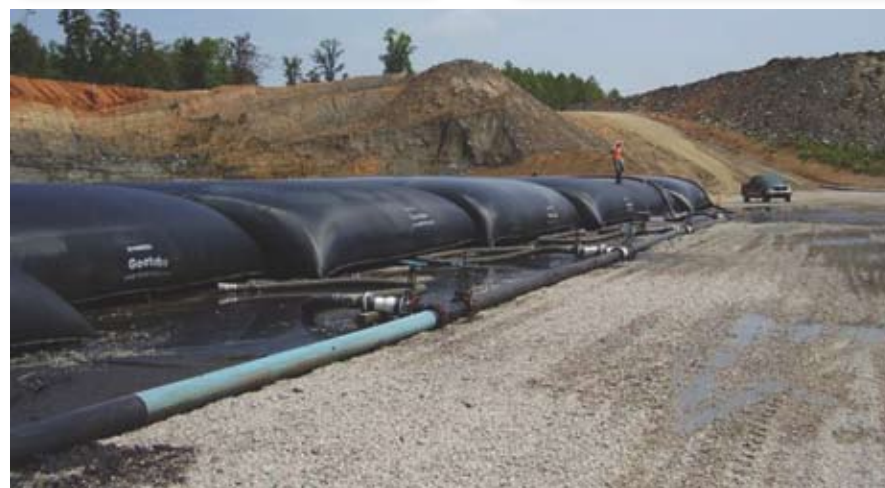
Geotextile tubes have a proven track record, and will retain sediments as water is drained into a collection system before routing to the water treatment plant.
