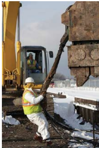
In 2007, Honeywell began building an underground steel barrier wall on the western shore of Onondaga Lake. Two phases of the barrier wall, which extends for 1.5 miles along the lakeshore, are complete. The wall blocks contaminated groundwater from old Allied Chemical properties in Solvay and Geddes from flowing or seeping into the lake.
