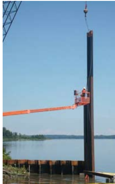
In 2007, Honeywell began building an underground steel barrier wall on the western shore of Onondaga Lake. Two phases of the barrier wall, which extends for 1.5 miles along the lakeshore, are complete. The wall blocks contaminated groundwater from old Allied Chemical properties in Solvay and Geddes from flowing or seeping into the lake.
