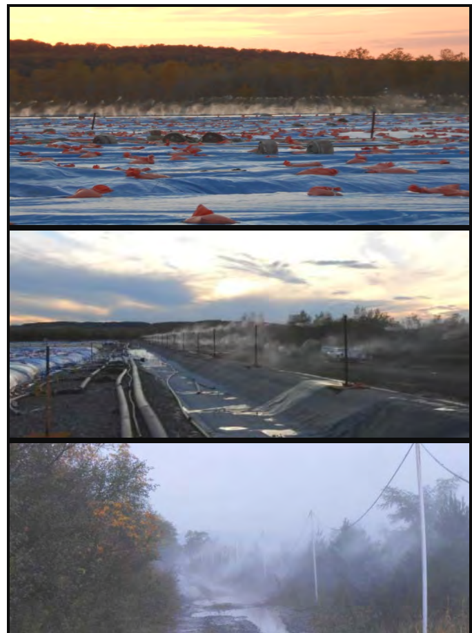
Misting systems throughout the site
