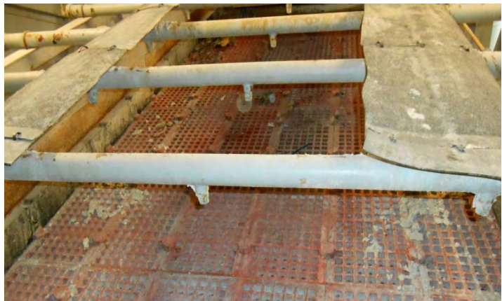
Debris water spray bars
