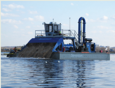
CAPPING 6,000 cubic yards of capping material placed.
