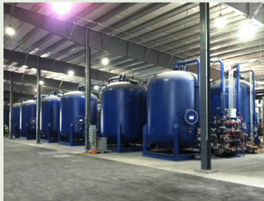
WATER TREATED Completed
