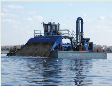
CAPPING 0 cubic yards of capping material placed.
