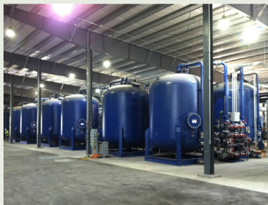
WATER TREATED Completed
