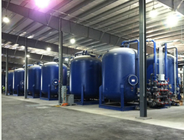
WATER TREATED Completed
