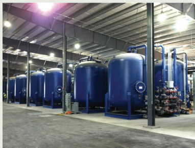
WATER TREATED Completed
