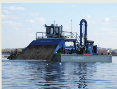
CAPPING 31,000 cubic yards of capping material placed.
