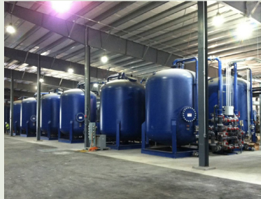
WATER TREATED Completed
