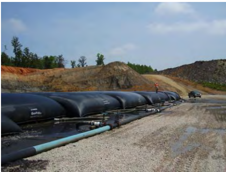
Geotextile tube dewatering operation
