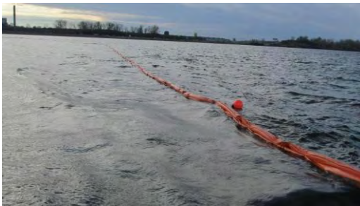
Silt curtain being deployed on Onondaga Lake.
