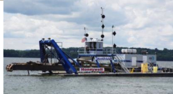
Work barges are clearly designated with proper navigational markings.
