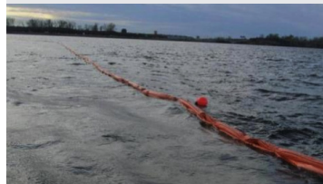
Silt curtains help control short-term impacts on water quality and keep lake material from spreading. Buoys are installed around activities outside of a silt curtain.
