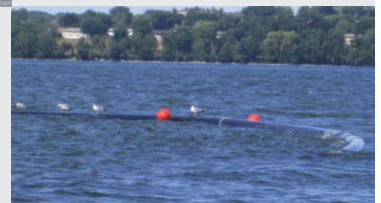
Silt curtains help control short-term impacts on water quality and keep lake material from spreading. Buoys are installed around activities outside of a silt curtain.
