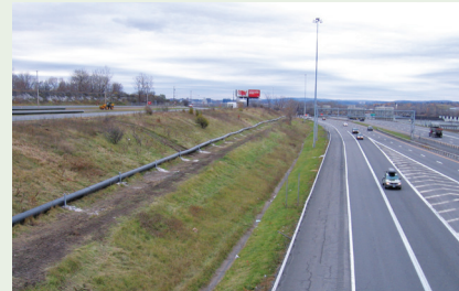
Sections of double-walled pipe connect to form the four-mile-long pipeline that transports dredged lake material.
