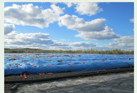
Dredged material is piped to the consolidation area.
