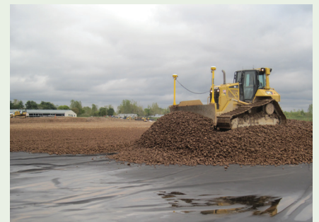
Gravel being placed on top of a high-strength liner at the consolidation area. Geotextile tubes are set on top of the gravel.
